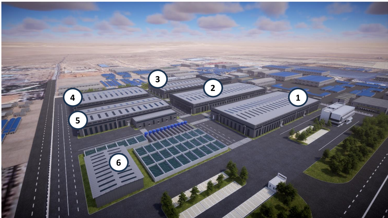
Note: 1. Spheroidization plant; 2. Purification plant; 3. Coating plant; 4. Finishing plant ; 5. Acid storage; 6. Water purification.
